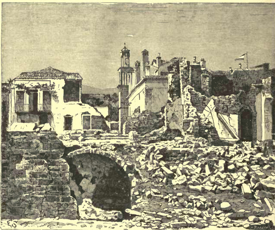
Fig. 136.—CHIO—VIEW TAKEN AFTER THE EARTHQUAKE OF 1881.
