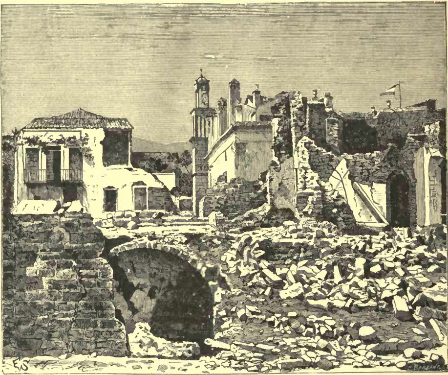
Fig. 136.—CHIO—VIEW TAKEN AFTER THE EARTHQUAKE OF 1881.
