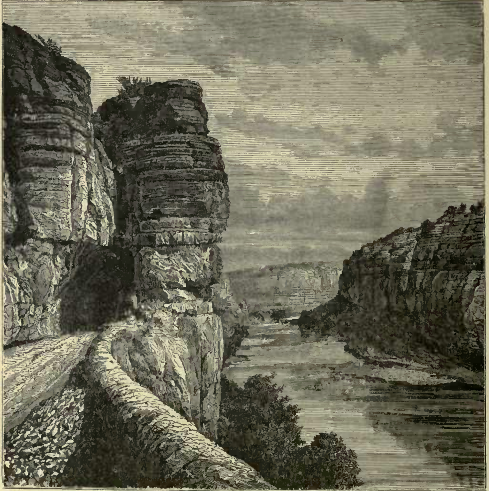
Fig 134.—THE DEFILE OF THE ARDÈCHE, NEAR ROOMS.
