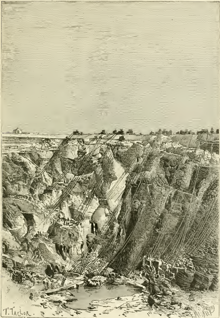
Fig. 47.—KIMBERLEY: APPEARANCE OF THE MINE IN 1889.
