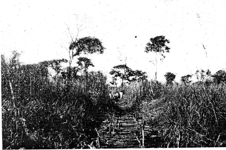
FIG. 8. LAMBA SWAMP BRIDGE
